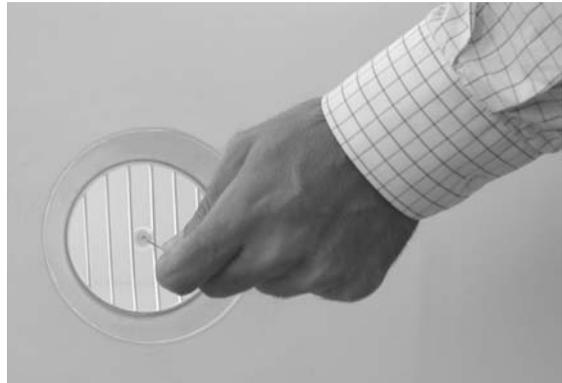
Tighten the cord and fasten it to the dent on the internal flanges.
