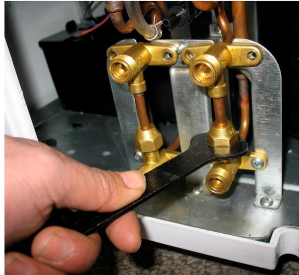
11. Fix the copper adaptors to the metal plate using the 4 screws then fix the flexible tube using the metal clip that you have taken off in the above step 8 (re. Pics 13 & 14)
